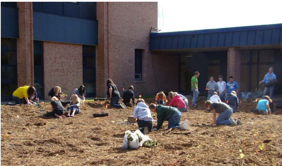
Installing a rain garden by the numbers: In three days more than 120 Fruitport Middle School students hauled 12 dump truck loads of dirt, spread 26 cubic yards of mulch, and placed 1,000 plants in their rain garden.
