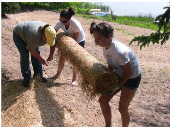
North Muskegon students installed mulch blankets to control erosion until their plants are established at Bear Lake.
